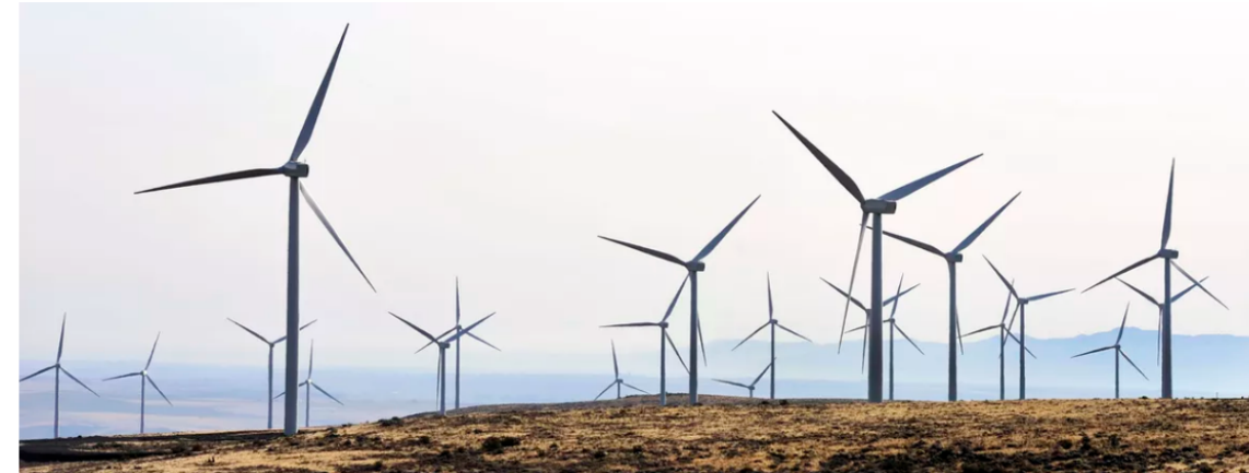
The view of the Wild Horse Wind Facility, Oct. 27, 2011, near Vantage, Wash. A proposed site combining wind and solar energy in South Central Washington is drawing a lot of attention from local residents (DAN PELLE)
